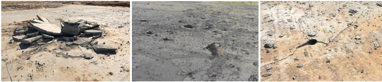
Figure 1: Image of crater (left), spall (middle), and camouflet (right).
